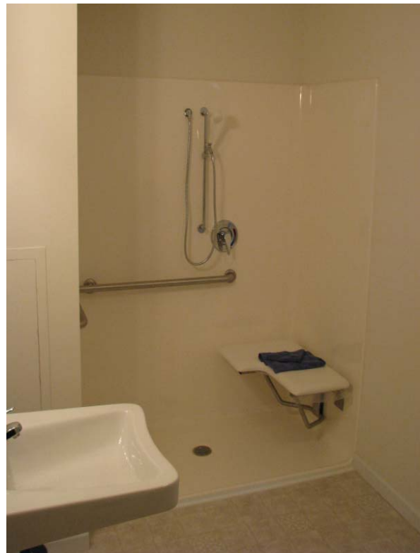
The home also includes a shower stall that can accommodate a disabled person. This bench allows a handicapped person to shower while sitting down.
