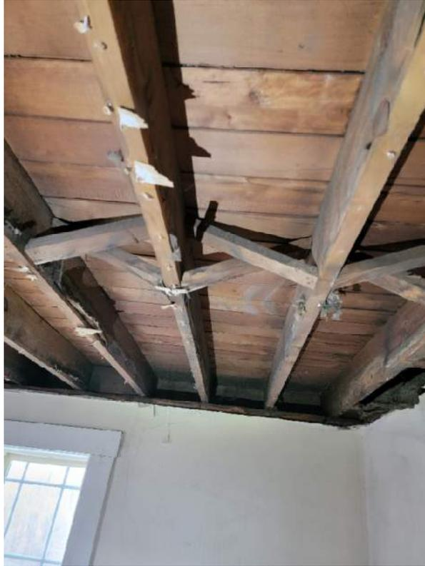
Joists showing nail pull over and nail withdrawal.
