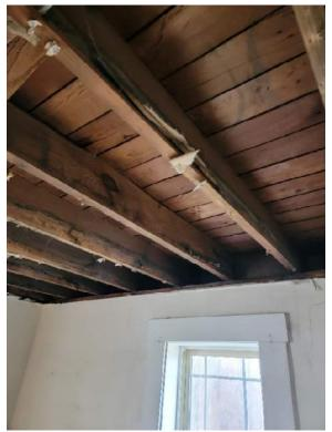
Joists showing nail pull over and nail withdrawal.
