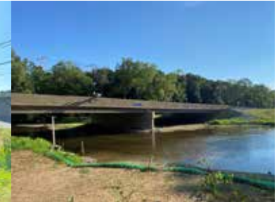
Completed bridge replacement on Rt. 322 (Downingtown Pike) crossing the Brandywine Creek.
